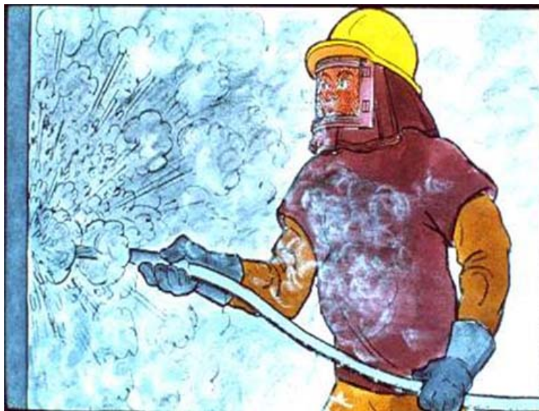
Figure 24. Sandblasting
